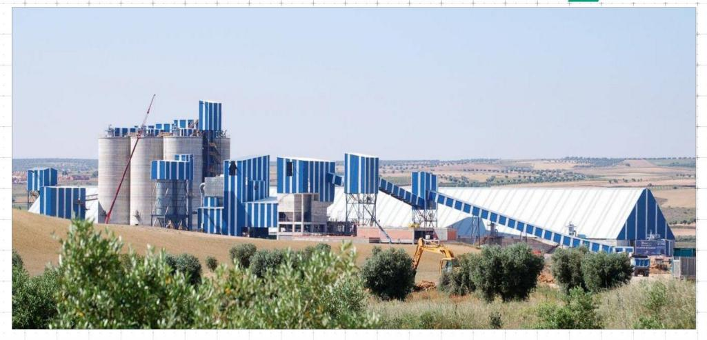
2006: EPC line 1, BM building. Storage silos, bulk load & packing. Capacities: 2 x 1.500 t/d
