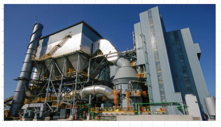
2014: Preassembled cement grinding station with MVR 5.250 kW, 210 t/h OPC. 3 x 200 t/h Ecohoppers; 90.000 Tm fully automated raw material warehouse. 7 x 3000 Tm cement/slag silos.
