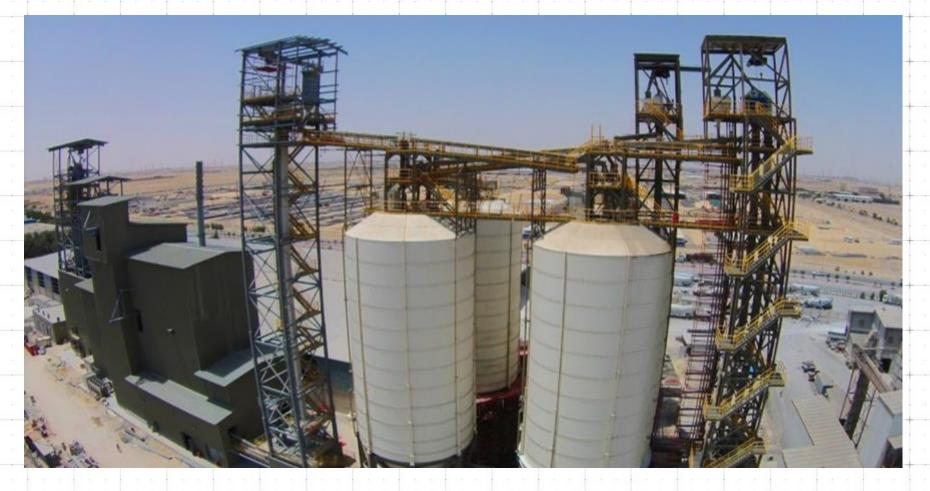
2015: Cement Mill 3. Raw material handling, ball mill house with Magotteaux XP4i classifier and silo feeding. Capacity: 3,000 t/d.
