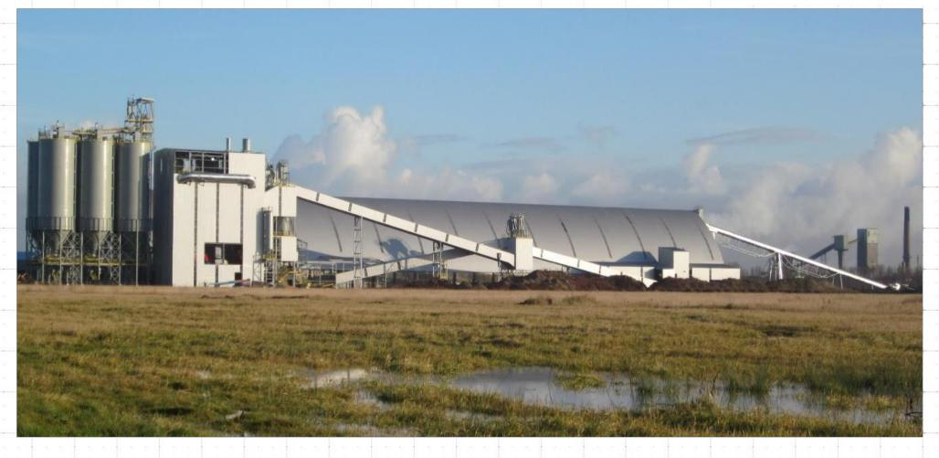
2012: EPC Cement grinding plant BM 110 t/h, 4.350 kW; including 6 x 3.000 Tm storage silos, bulk loading and packing unit.
